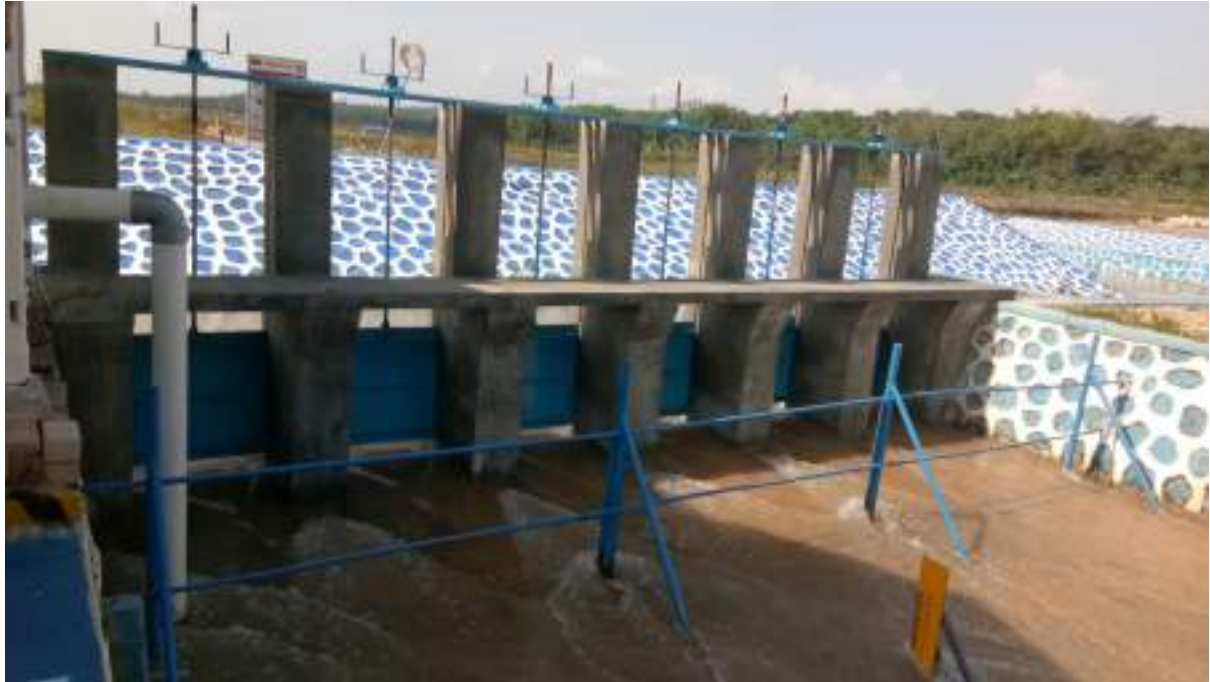
Settling Pond PT. Adaro Indonesia, lokasi: Tutupan
