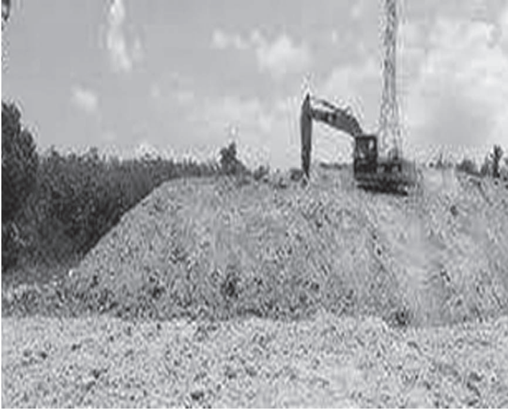
Gambar 2.3 Metode Controlled Landfill
